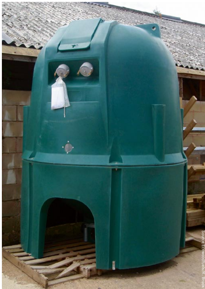
External pellet fuel store, similar to external oil tank. Capacity 1.5 tonnes.
