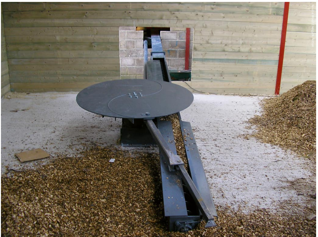
Fuel store agitator, pressure plate and in-feed auger.
