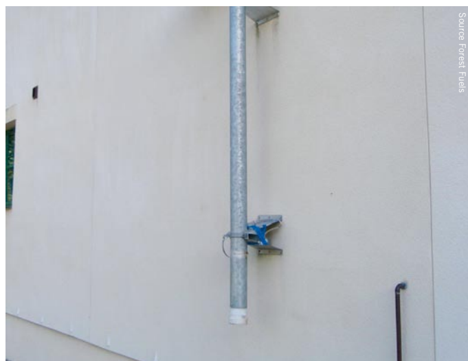
Feed pipe and nylon coupling for blown pellet deliveries direct into the fuel store
