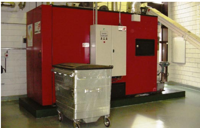
Compote Compact C70DHV Boiler 700kW
