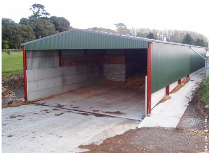
Warehouse size fuel store and boiler house walking floor and ram fed fuel delivery mechanism – capacity 500 cubic metres – annual usage 8–10,000 cubic metres.
