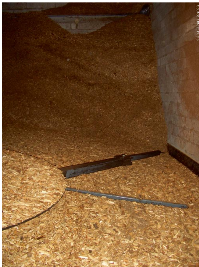
Dead space within the fuel store inaccessible corners beyond the range of the agitator
