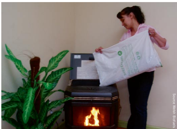
Pellets being poured direct into the fuel hopper of a room heater
