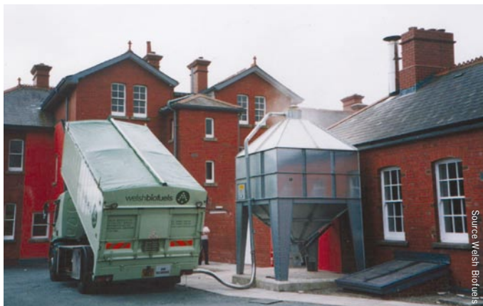
Blown Pellet Delivery – Note dust emerging from vent at the top of the store helping to depressurise the store during delivery
