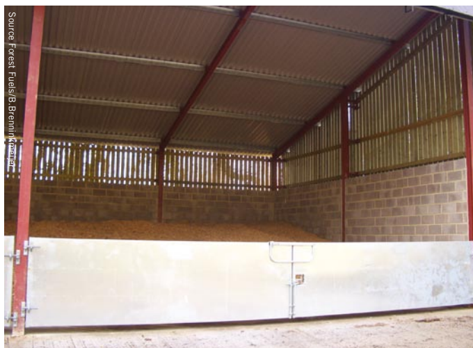
Well designed fuel store built to an Austrian specification–power floated concrete floor, good ventilation, excellent access for haulage vehicles and chipping, reinforced pushing wall, rear of structure orientated towards prevailing weather conditions.
