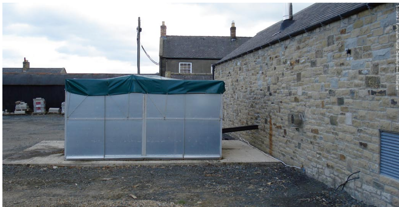
Low cost galvanised woodchip store suitable on agricultural site where machinery is available to permit loading
