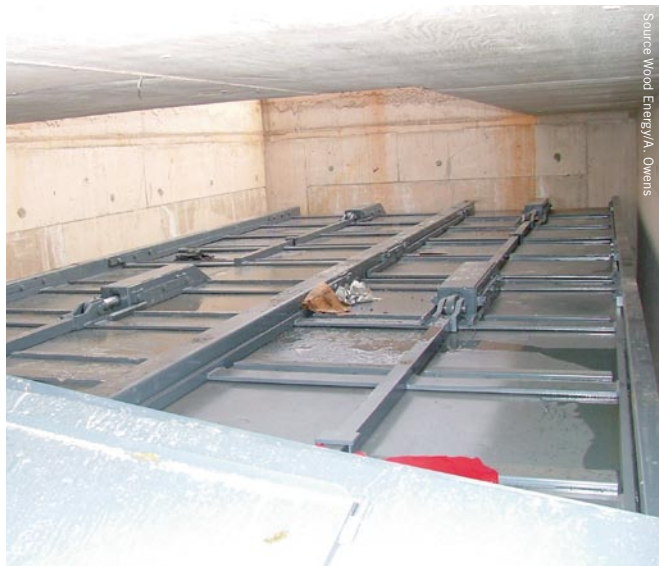
Walking floor mechanism prior to installation
