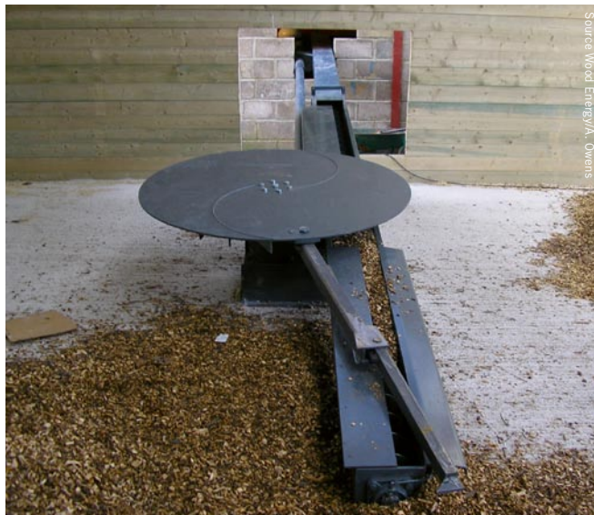
Fuel agitator and pressure plate Empty
