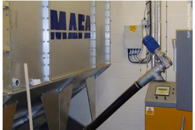
Galvanised pellet store, pneumatic delivery via inlet pipe from building exterior
