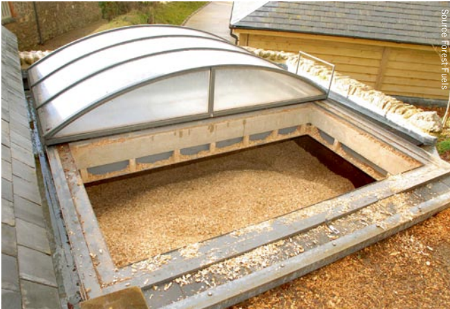
Well designed subterranean fuel store for woodchip permitting tipped delivery – sliding roof cover
