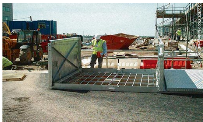
High quality fuels store, metal safety grid, “book” opening doors prevent tipped fuel spilling
