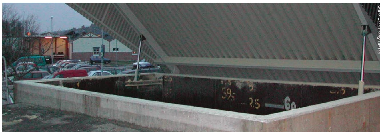
Hydraulic lid has insufficient lift to permit easy tipping and no safety bar in place to prevent reversing vehicle contacting the edge of the fuel store
